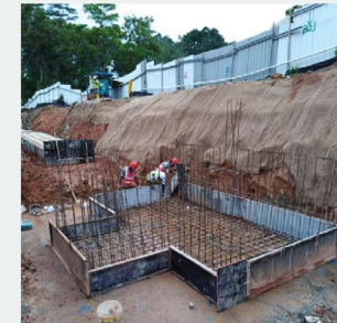
Underground Electrical & telecom Lead-in Pipe works: Concrete haunching of pipes in progress
