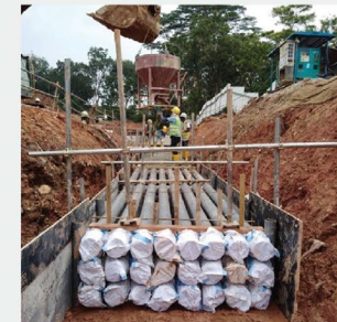
Underground Electrical & telecom Lead-in Pipe works: Concrete haunching of pipes in progress
