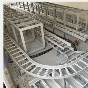
Our team successfully installed cable ladders as supports for high-volume or heavy cabling.
