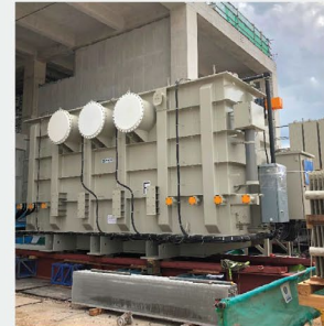
230kV 150MVA Transformer Installation
