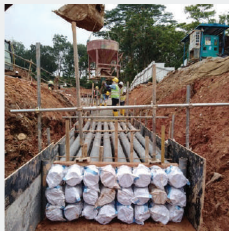
Underground Electrical & telecom Lead-in Pipe works: Concrete haunching of pipes in progress
