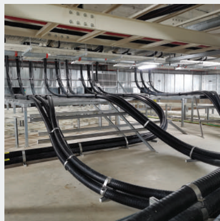
230kV Cable Installation
