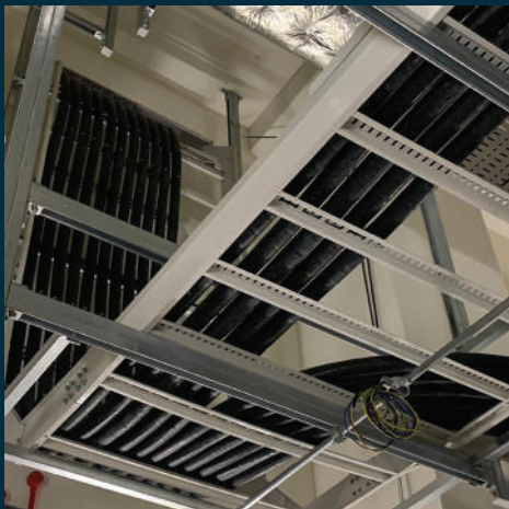
Successful installation of the HV 12.7/22kV cable on the cable ladder system.
