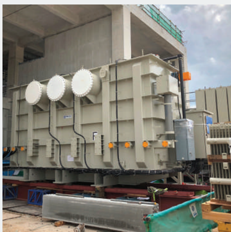
230kV 150MVA Transformer Installation
