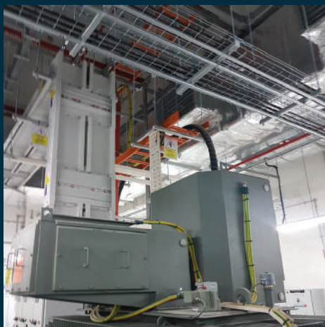
Electrical Power Distribution Network & Cabling Works - Indoor busducts & termination work to transformer, cable containment & cabling works
