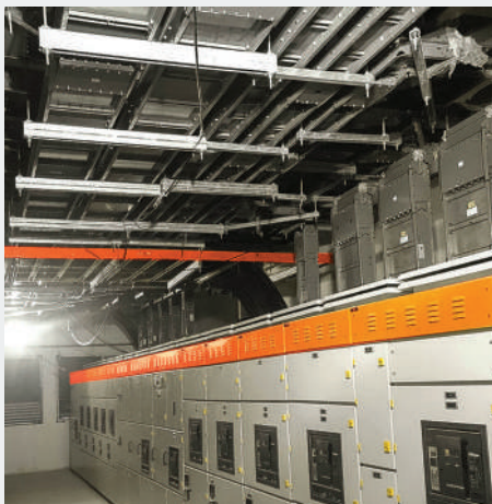
Busduct connection to switchboard
