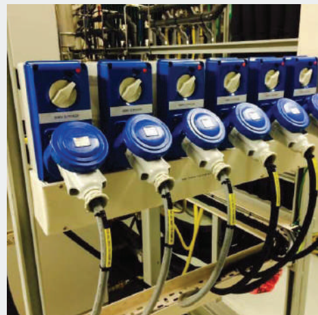
Supply & Install LV Provision of CEE FORM for hook-up of wafer-chip Fabrication
