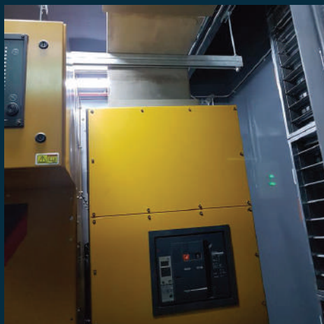
Electrical Power Distribution Network & Cabling Works - Cast resin busducts & termination work inside generator enclosure
