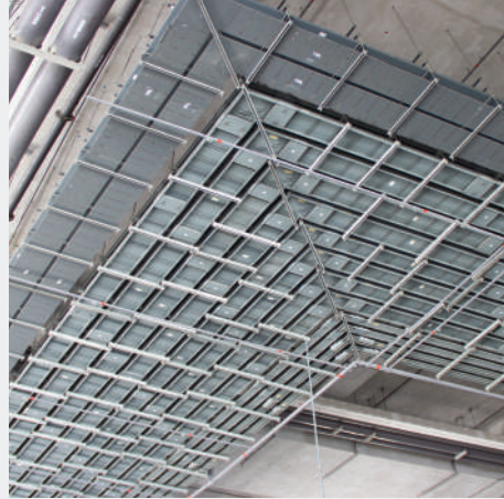
Securely mounting busducts to unistrut supports and aligning ends of adjoining sections.
