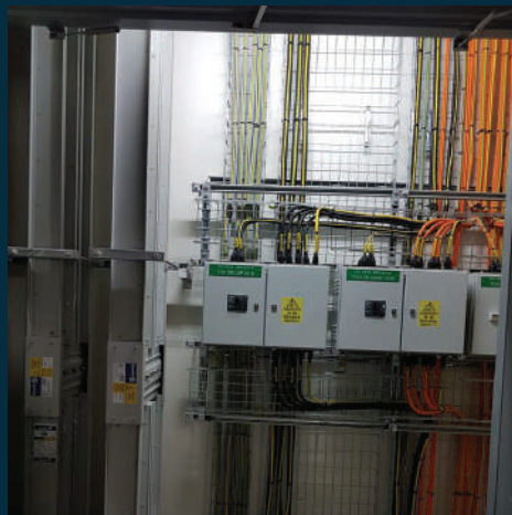
Electrical Power Distribution Network & Cabling Works - Work Done in Electrical Riser
