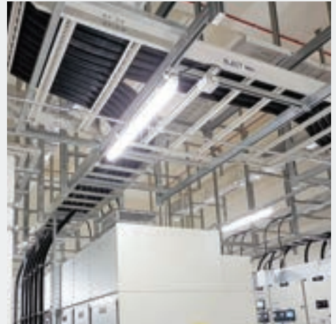
Completed installation cabling work to the switchgear panel
