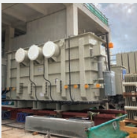
230kV 150MVA Transformer Installation
