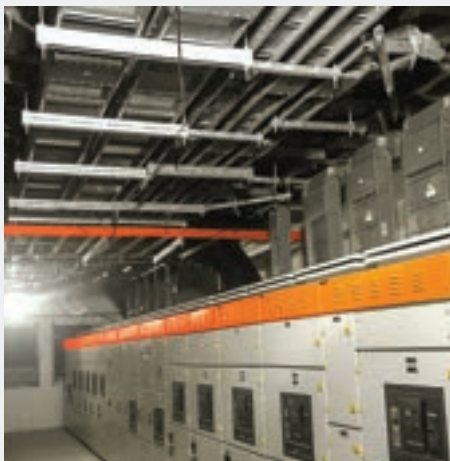
Busduct connection to switchboard
