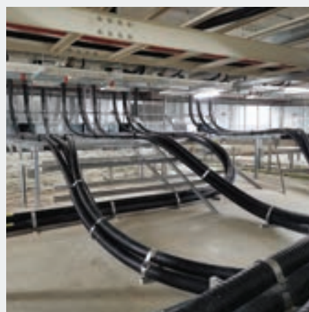
230kV Cable Installation
