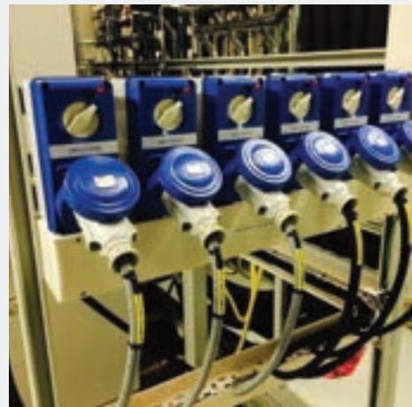
Supply & Install LV Provision of industry socket (Ceeform) for hook-up of wafer-chips Fabrication
