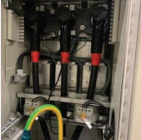
Completion of termination work for 22kV at the switchgear was a critical milestone in the project
