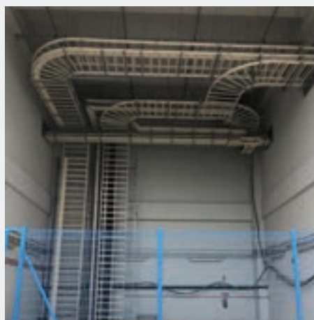
Cable Support Installation
