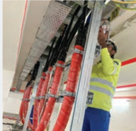
HV cable at the substation cable chamber room, ensuring the proper functioning of the high voltage cabling system
