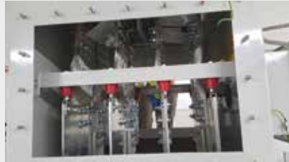
Supply and installation of busduct termination within the transformer
