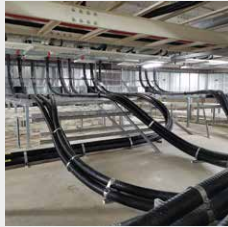
230kV Cable Installation
