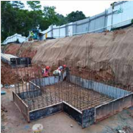
Underground Manhole: Cast-in Situ Work in Progress
