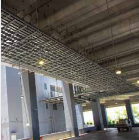
Mounting busduct on supporting brackets at ramp up drive way.
