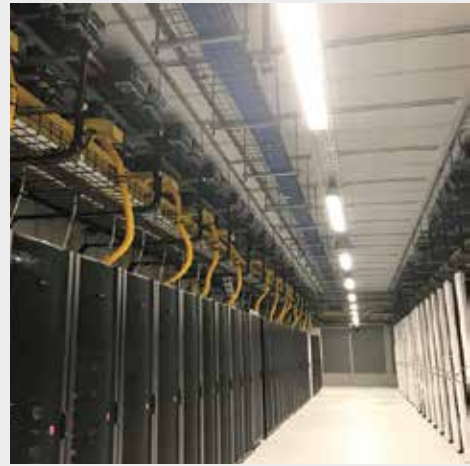
Distribution Busducts Installation in Data Hall
