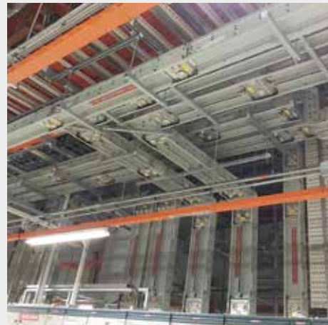
Supply & Install of MV/LV Busducts for control panels & Load Centre
