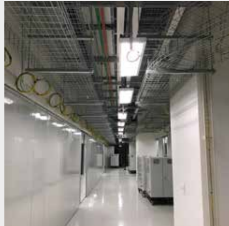
Customised metal fabrication works - cold aisle installation using hollow sections & unsaturate
