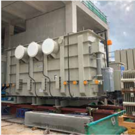
230kV 150MVA Transformer Installation
