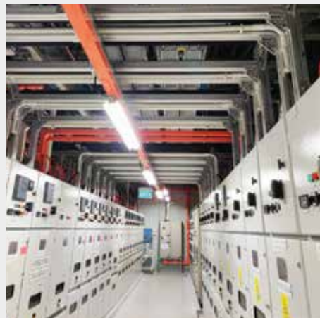
6.6kV Busducts Installation
