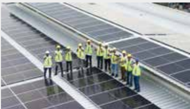
Successful Solar Photovoltaic (PV) Installation at B'EV Terminal Charging Hub
