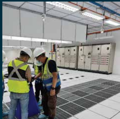
Data Centre Construction Air Balancing Testing
