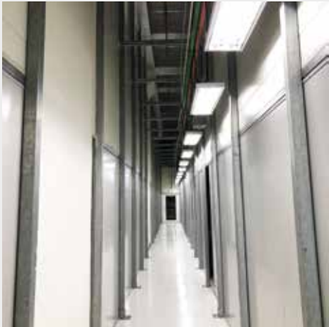
Customised metal fabrication works - hot aisle installation using hollow sections & unsaturate
