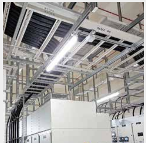
Completed installation cabling work to the switchgear panel
