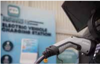
Successfully installed the 22kW AC charger at Busways Headquarters
